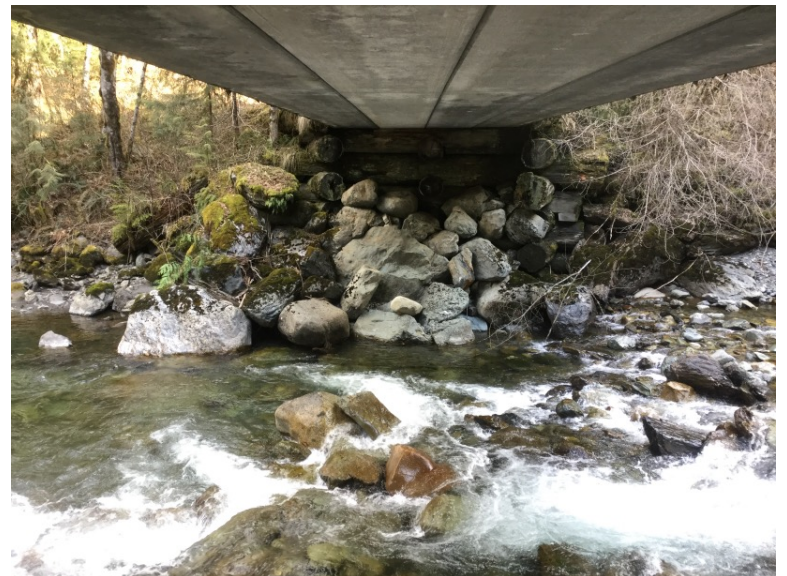
Right Bank Abutment when facing downstream
