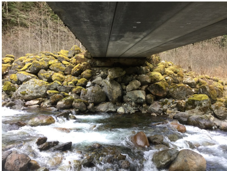
Left Bank Abutment when facing downstream
